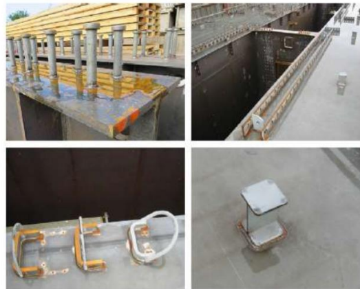
Fig.5:-Typical shear connectors
