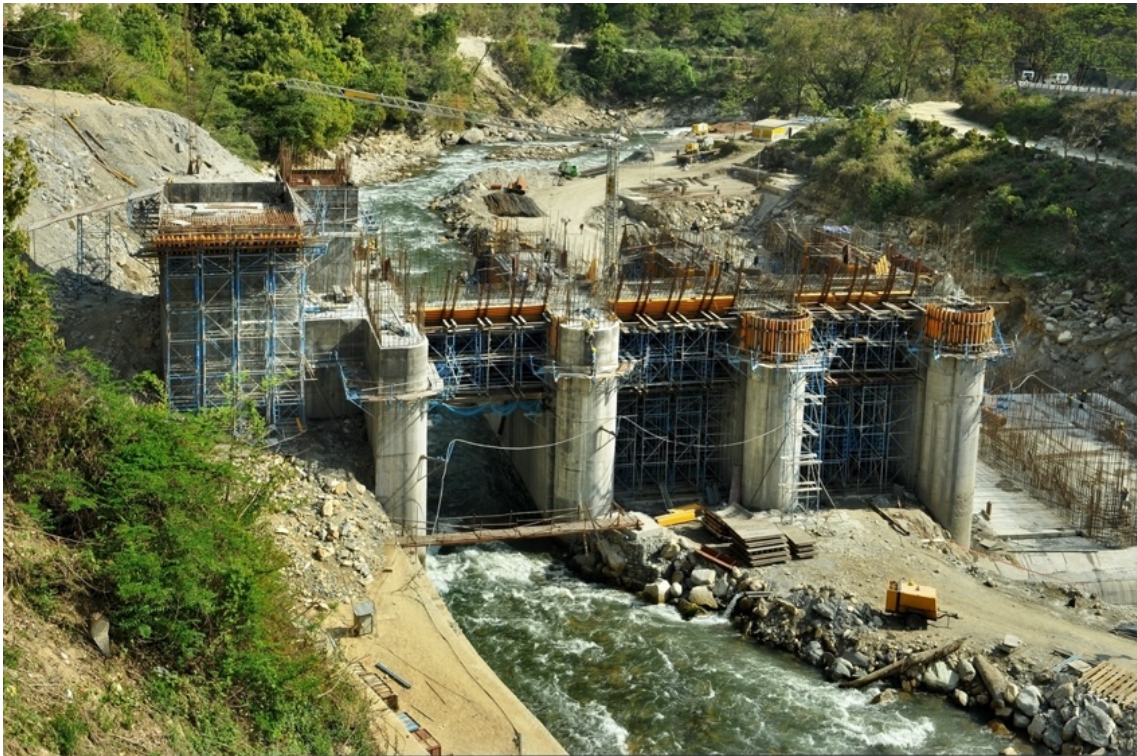
Figure 3.13 Construction site of a hydropower project in Nepal (Source: orin/shutterstock.com)
