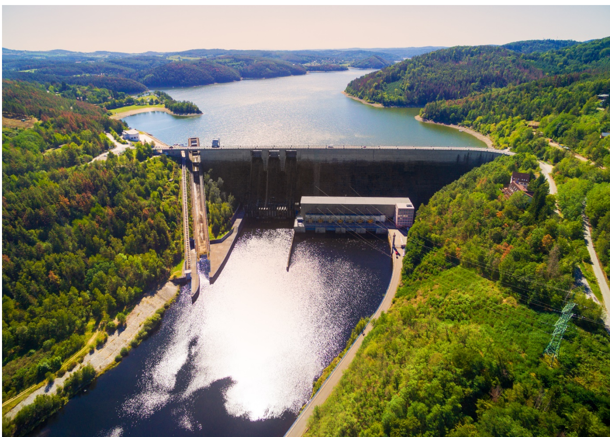
Figure 3.5 Impoundment area for hydroelectric production (Orlik Reservoir, Czech Republic) (Source: Kletr/shutterstock.com)
