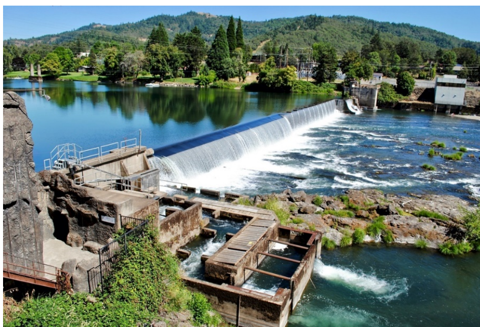
Figure 4.1 Fish passage facility at the right riverbank of the Winchester Dam, Oregon, in the U.S.
