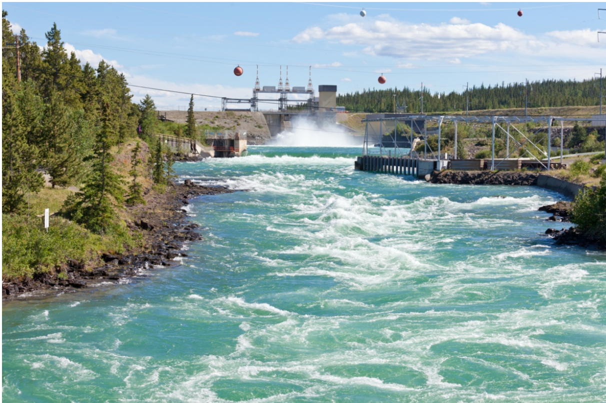
Figure 3.10 Near-surface supersaturated “white-water” release from small-scale HPP in Canada (Source: Pi-Lens/shutterstock.com)
