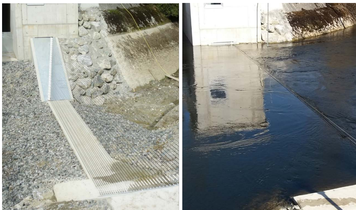
Figure 4.18 Illustration of hybrid barriers to guide the fish to a nearby bypass (visible in the upper left corner). The horizontally tensioned steel cables only serve to protect fish and can be completely laid down on the riverbed for cleaning and flood discharge (Source: Markus Auflager)
