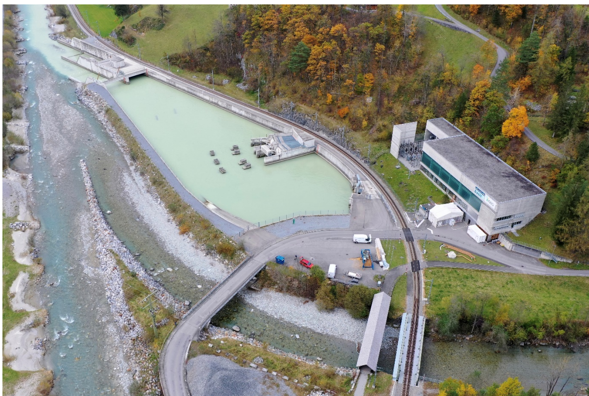
Figure 4.29 Drone footage of a retention basin with energy breakers in Switzerland, designed and operated to dampen hydropeaking waves (Source: Reuther Kristof)
