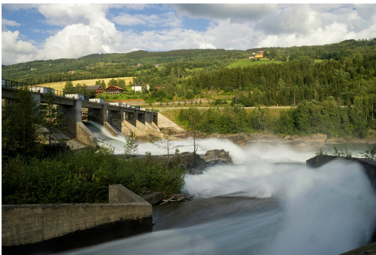
Figure 2.1 Spill over run-of-river hydropower dam at Hunderfossen on River Gudbrandsdalslågen, Norway (photo credit: jstuij/shutterstock.com)
