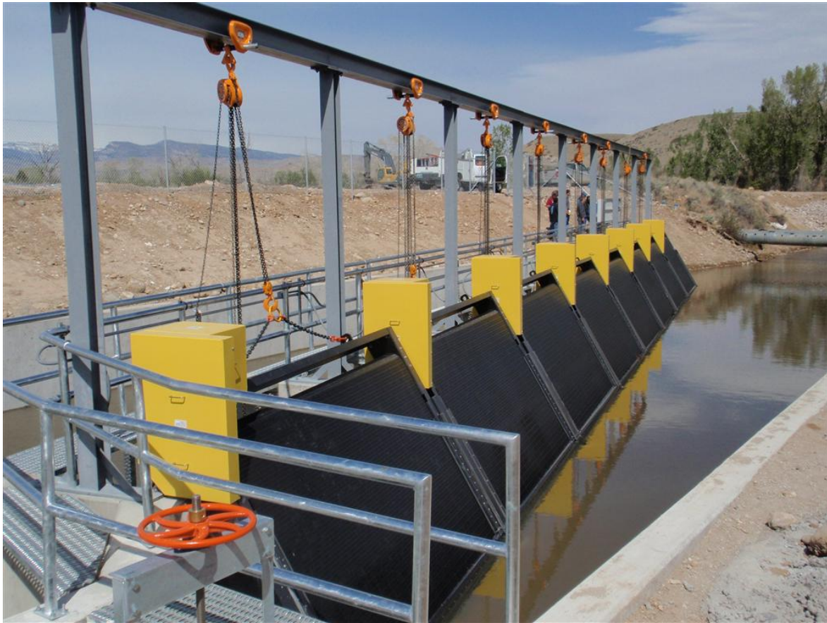
Figure 4.12 Vertically inclined flat plate at the Little Wind River in Wyoming, USA
