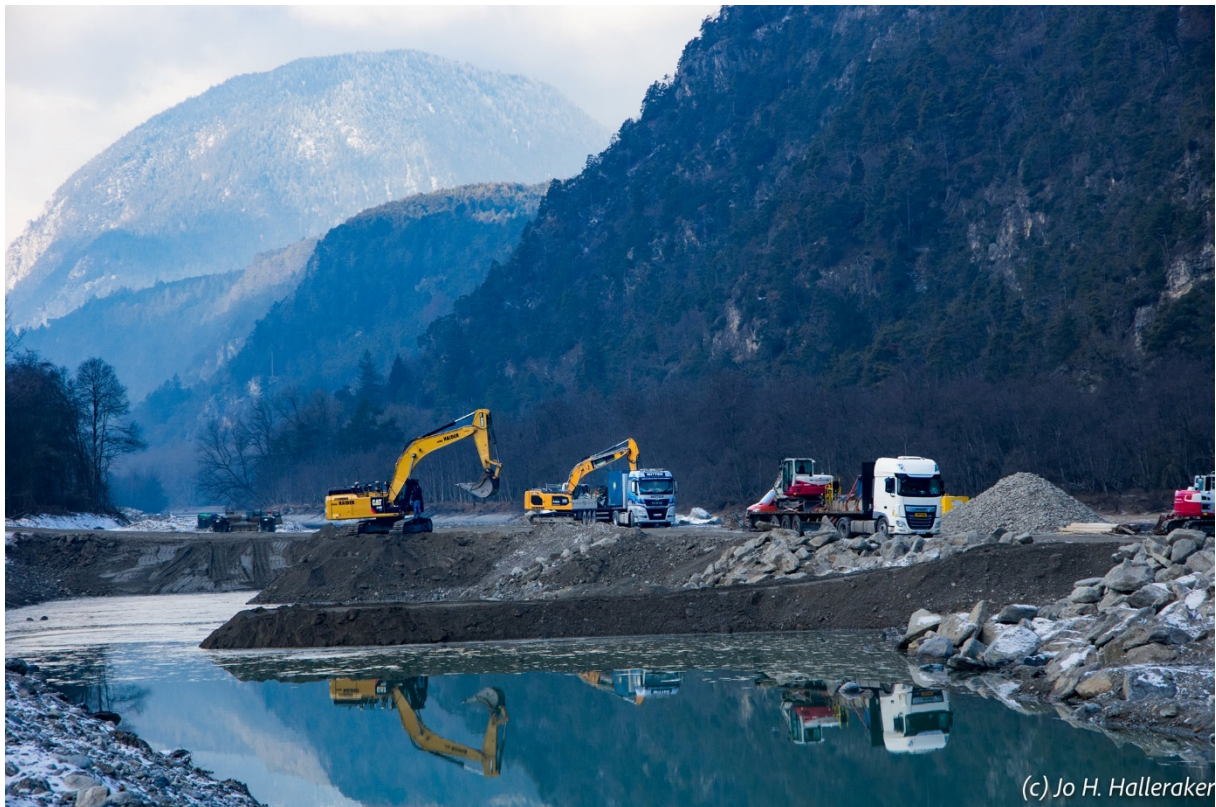
Figure 4.30 Example of compensation measures in the Alps: river widening by reallocating embankments and restoring gravel bars in River Inn, Austria, to reduce the cumulative impact on fish communities in River Inn, financed by the hydropower plant owner. (Source: Jo Halvard Halleraker)
