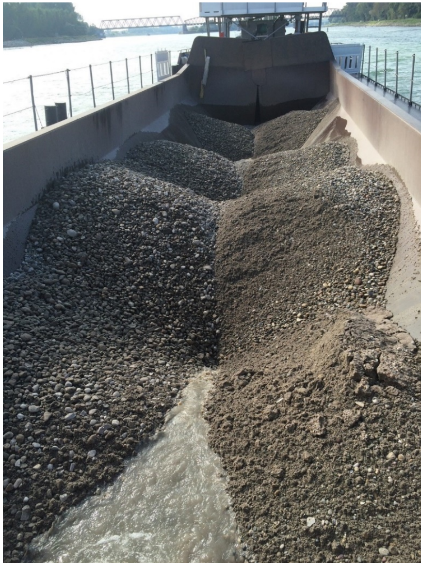
Figure 4.22 Process of sediment feeding on the River Rhine (Source: Marcell Szabo-Meszaros)
