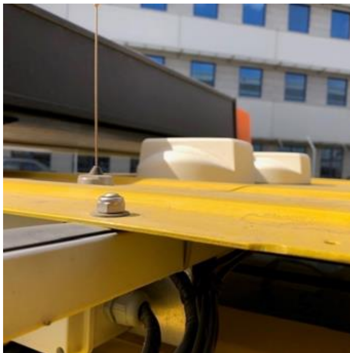
Figure 24. Follow-me LTE antenna installation
