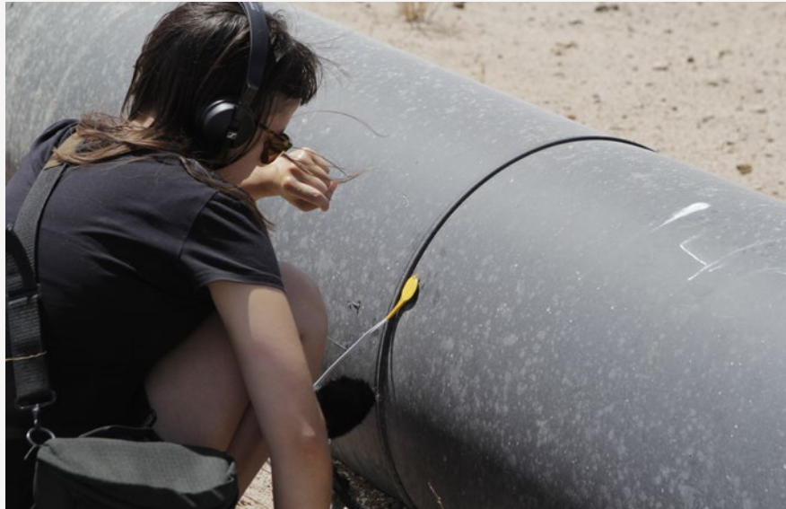
Daniela using a mic contact for recording the sounds of the water running through a pipe used for lithium extraction. Image credit: Josefina Buschmann.
