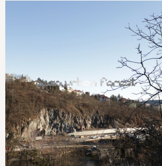
Construction site facing the forest across the river, opposite the Open Urban Forest garden. Image credit: Michal Mitro
