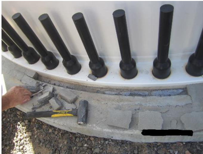
Grout Failure
