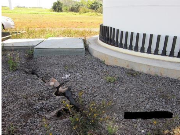
Geotechnical Failure
