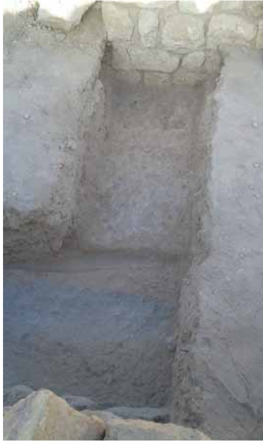
US846 floor with drain channel US847
