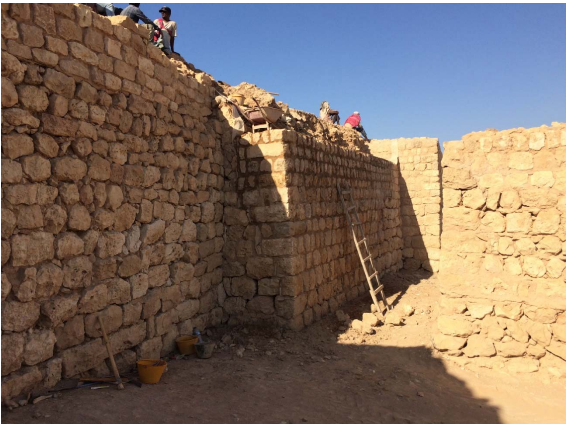
On 28 th November 2015, the wall was as shown below.
