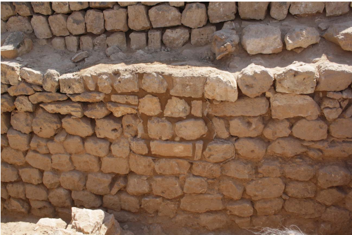
M555 after restoration
