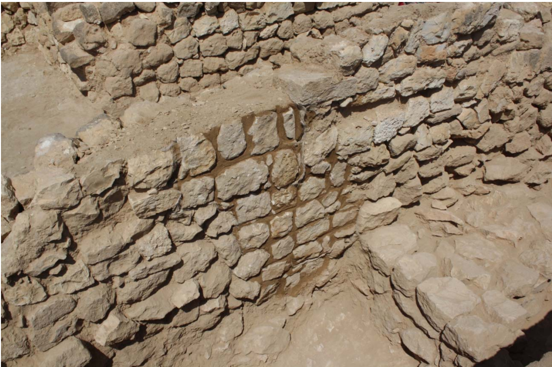
M550 after restoration
