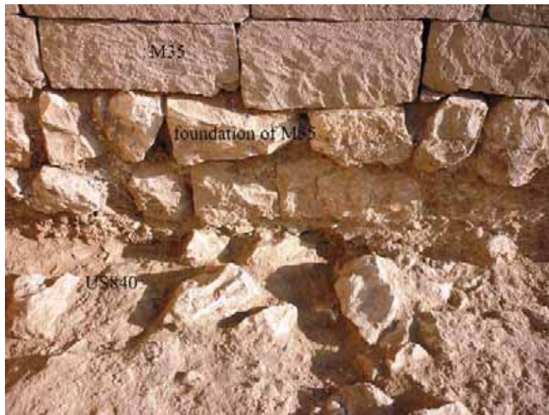
Particular of foundation of M35
