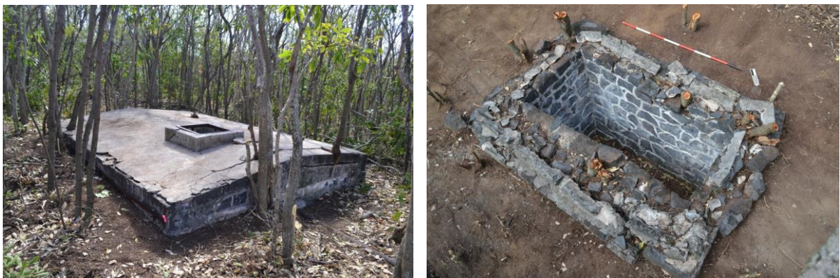
Figure 7. The water cistern and the underground storage room at Hospital 2.
