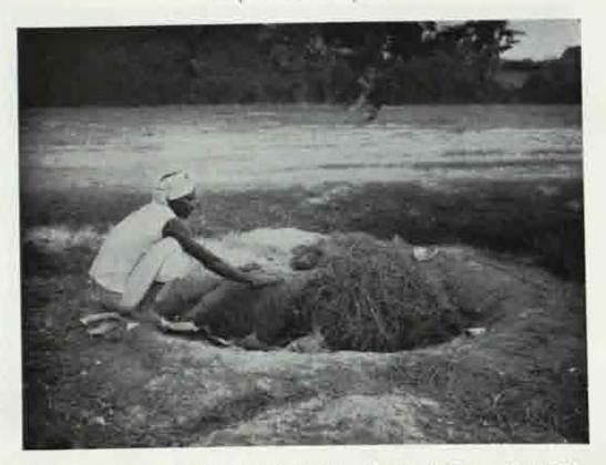
B. Lausadiya: potter applying a thin clay-coat over the shroud of straw. See p. 252
