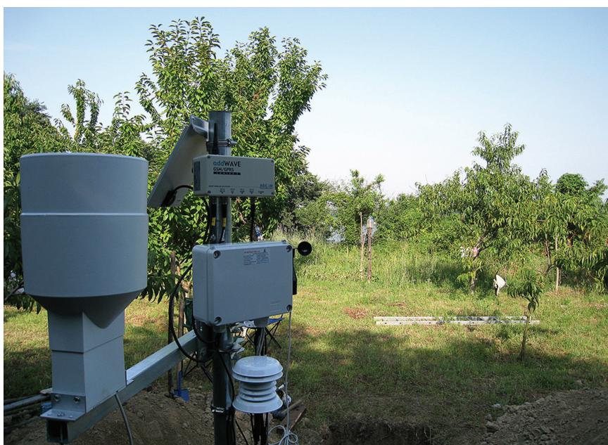
Fig. 1. General overview of the weather station at the study site.
