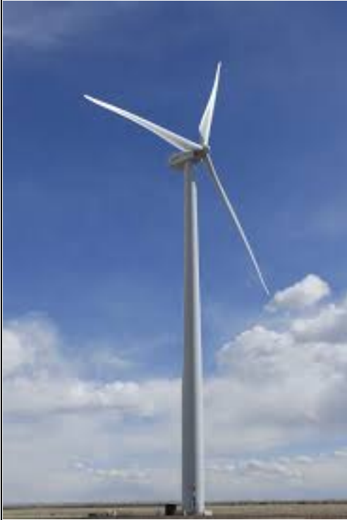
Figure: Onshore 1.5MW wind turbine (picture by Jeroen Van Dam NREL)
