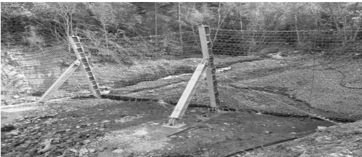
Figure 1. Debris protection devices
