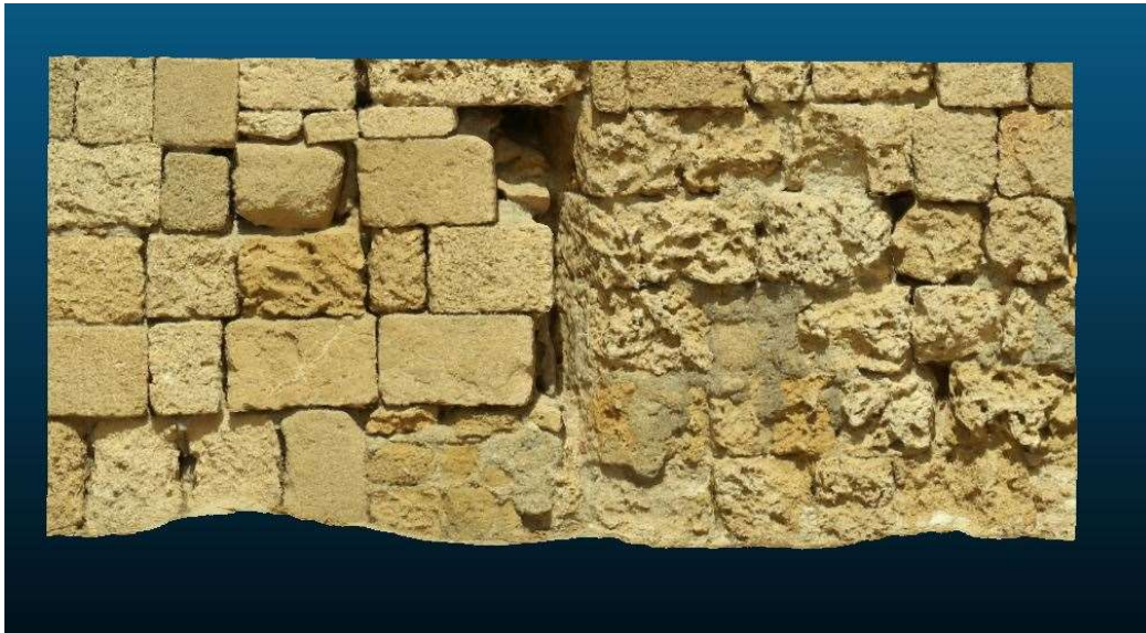
Figure 44: The Detailed 3D Textured Model where the erosion is obvious at specific stones.
