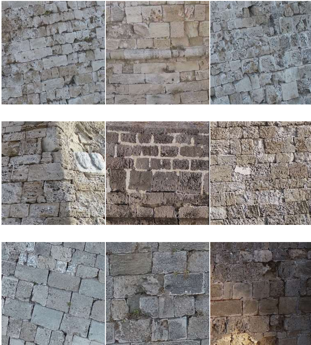
Figure 50: Images of the sites with No Cracks.
