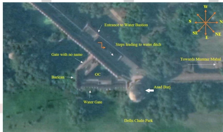
Figure 2: Google earth 3D view of south east corner of Red fort. Barican enclosing triangular outer courtyard (OC).
