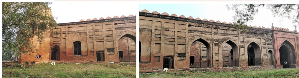
Figure 6. Terrace view of Asad Burj
