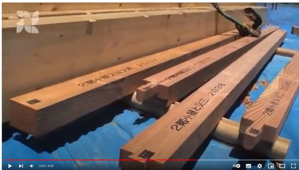
Figure 2. Individual beams of the ‘Onjuku Beach House’; Well visible: the machine-made joints (csxlab, 2012)
