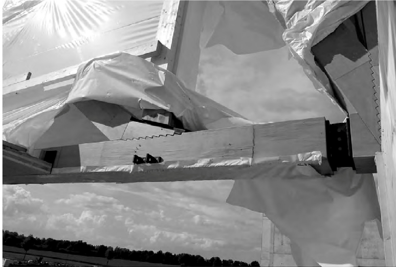
Fig. 3: Timber frame knot with 'zig-zag' joint [Hermann Kaufmann + Partner ZT GmbH n.d.].
