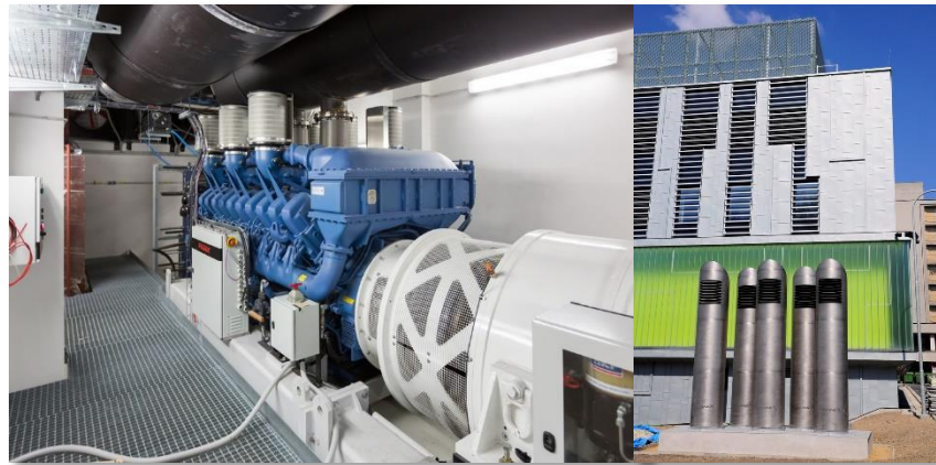
Dynamic rotating UPS 2x2,5MVA
