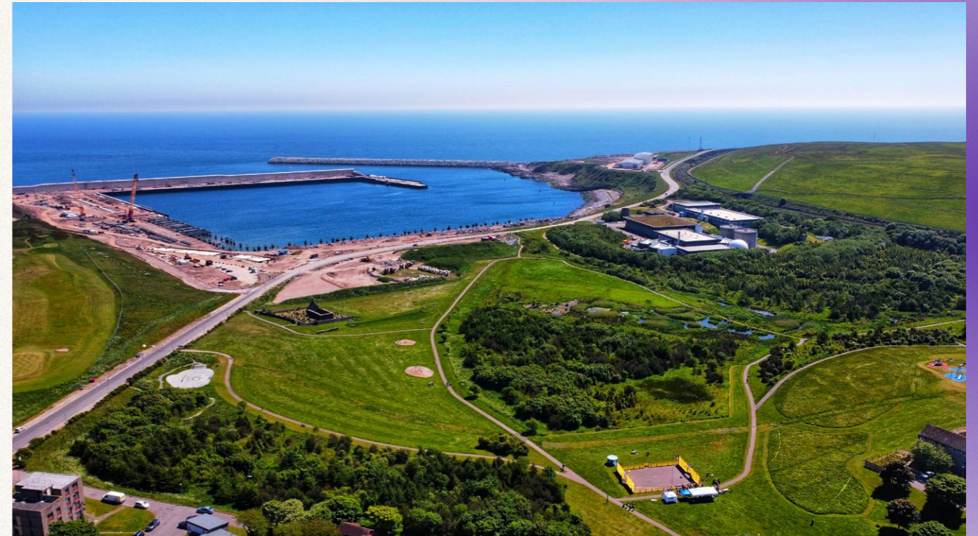
St Fittick's Park. Photo: Natalie Hood.
