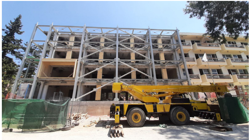
ProGETone demonstration project in Athene, seismic proof renovation
