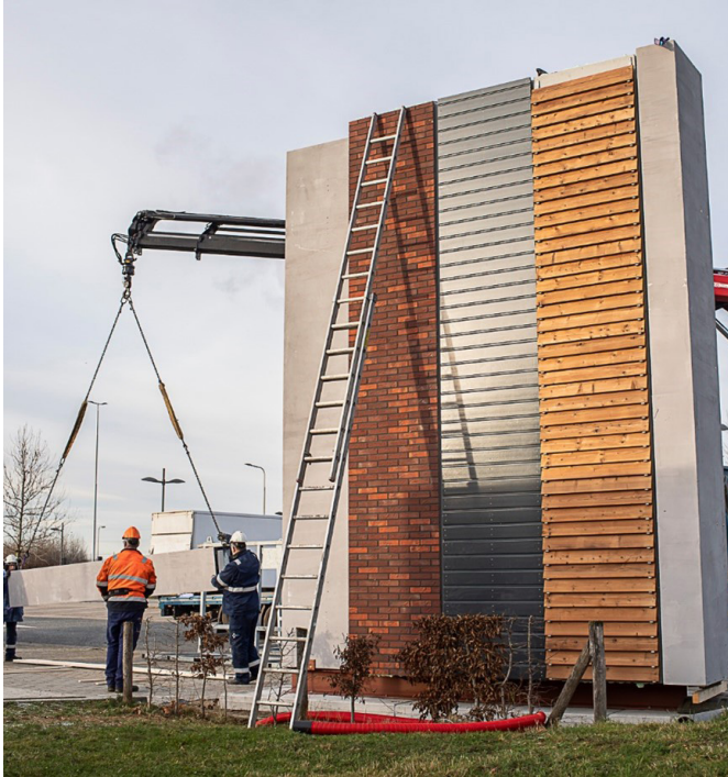
Left - Example of a modular and industrialized Building Envelope Kit from the DRIVE 0 project
