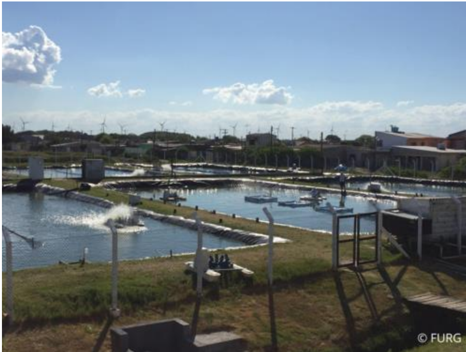
Figure 5. A mechanical aeration system in operation in the shrimp ponds at FURG, Brazil
