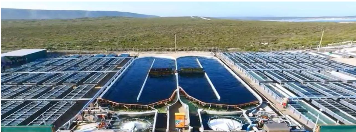
Figure 3. The Buffeljags abalone farm IMTA system, part of the South African IMTA lab, with seaweed ( Ulva ) raceways in the center and the abalone tanks on the sides. The Ulva oxygenates the water, absorbs CO 2 , and takes up ammonia so that the water can be safely recirculated back to the abalone raceways (credit: Viking aquaculture)
