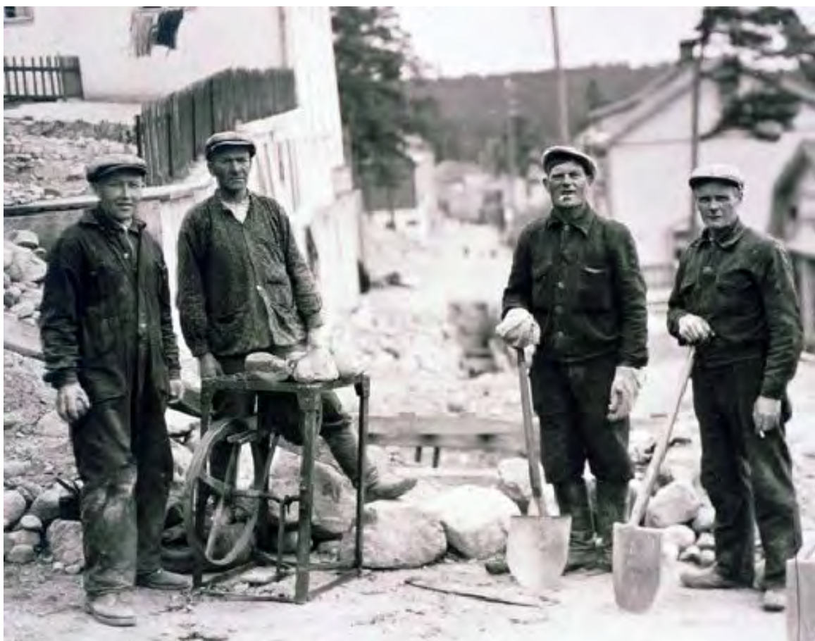
Picture N° 2. Installing the water mains.
