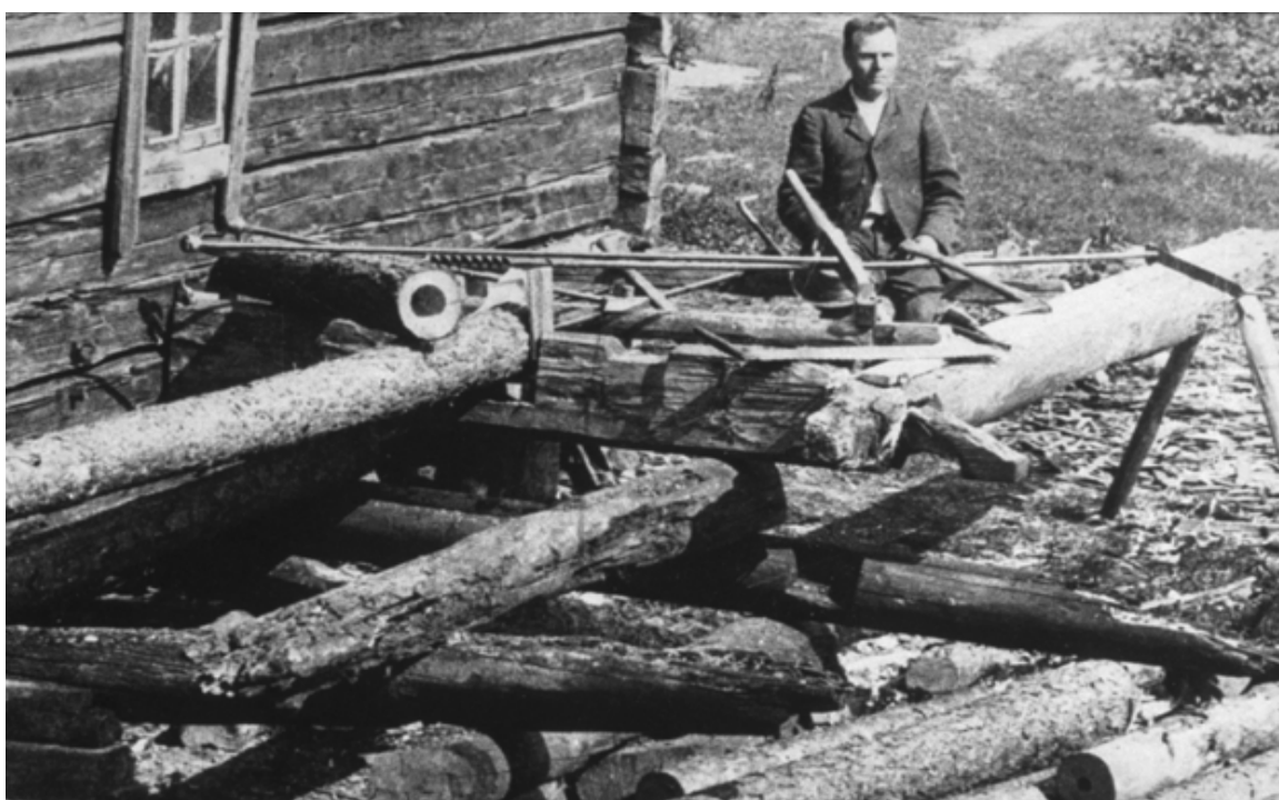
Picture N° 1. Drilling of wooden water pipes in 1913
