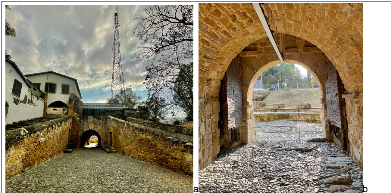
Figure 2.2 - Paphos gate: a) internal access of the Gate and b) the survived door (@authors)
