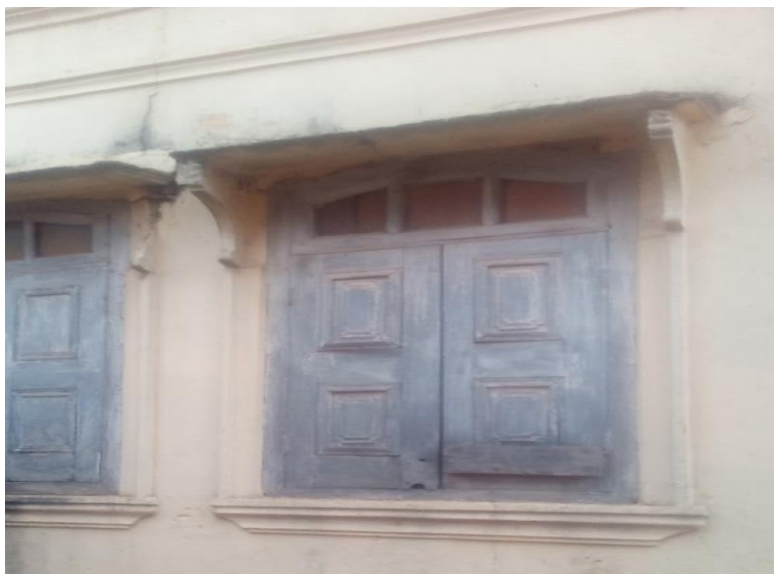
Plate 6: Exterior window with hood
