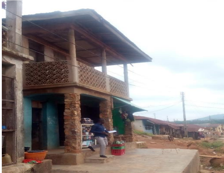
Plate 3: A vernacular building with roof eave building projection to protect the building from weather conditions.
