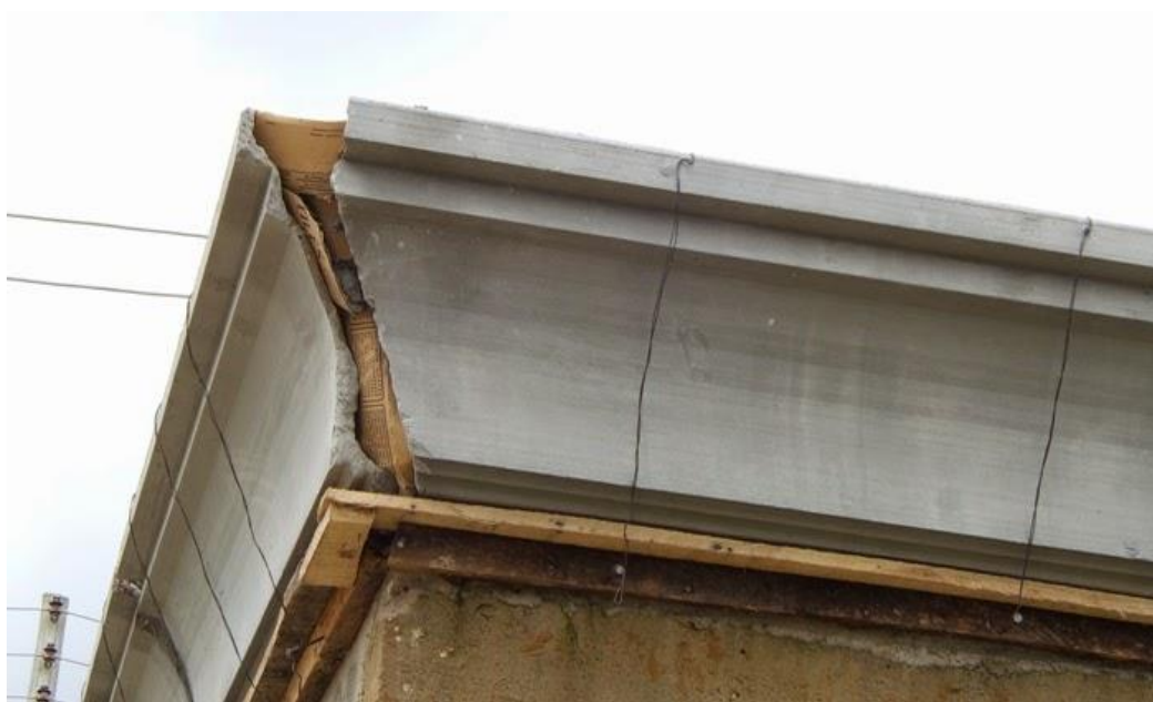
Plate 2: Concrete fascia element of contemporary residential building; exposes the walls and windows to adverse weather conditions . Source: Spydercraft (2015)
