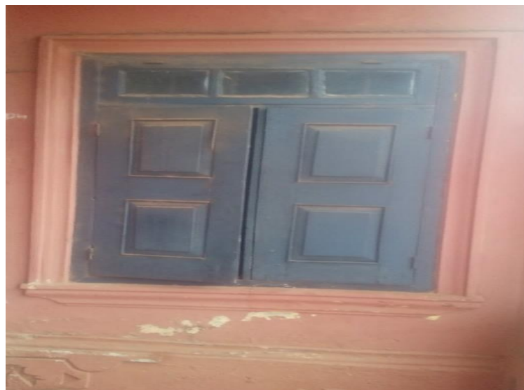
Plate 4: Casement window of Vernacular that allows for maximum ventilation compared to contemporary sliding windows.
