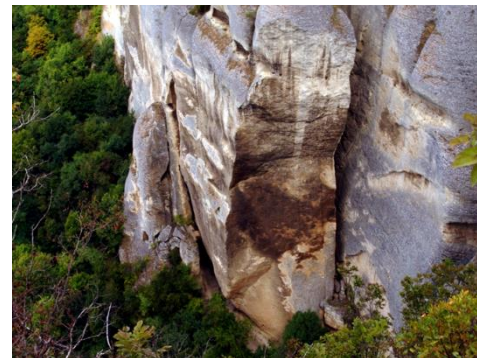
Figure 11. Landslip in front of the entrance to the Nimfite cave
