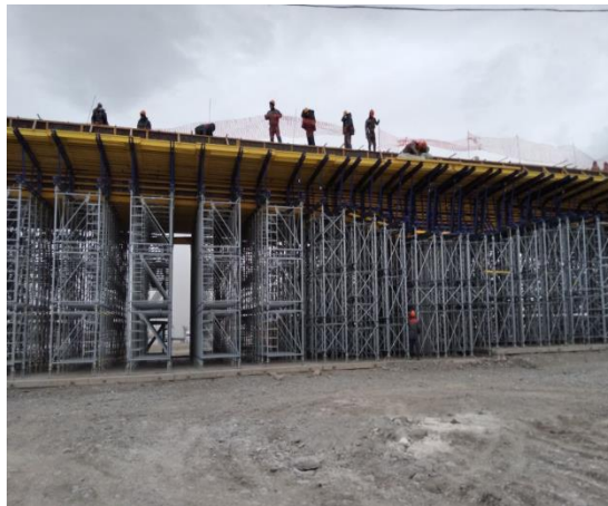
Fig. 10. Construction of span structures: a, b, c - special auxiliary structures and devices for the construction of a span structure; d - view of the overpass after completion of construction in Samarkand
