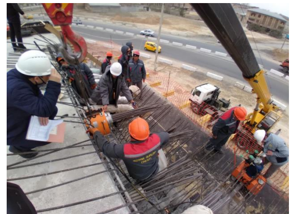
Fig. 11. "Post tension" - further tension
