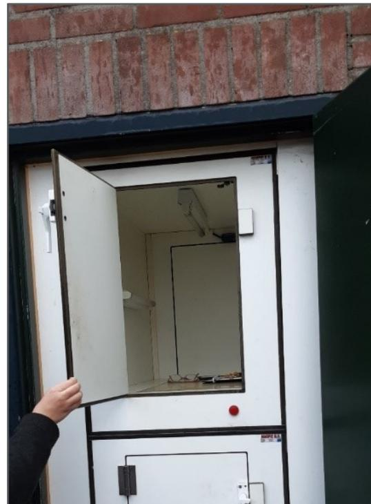
*Picture: A UV-decontamination chamber for personal items or equipment. The items can be retrieved after the procedure from the inside of the building.*
