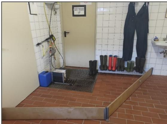
*Picture: This image shows an example of a boot cleaning station with a cold-water high pressure cleaner and a hygiene lock demarcation on the ground. The demarcation provides a physical barrier between the cleaning station and the outside area. An elevated stack for the cleaned boots enables any dirty water to run away whilst the boots dry.*
