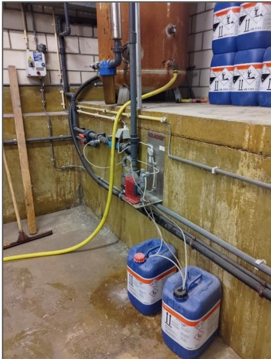
*Picture: This image shows an example of how to reduce the risk of contaminated water entering the pens. Here we see the equipment used for cleaning and disinfecting the drinking water system. The chemicals used to clean the system are stored appropriately and should be checked regularly for any signs of leakage or damage.*
