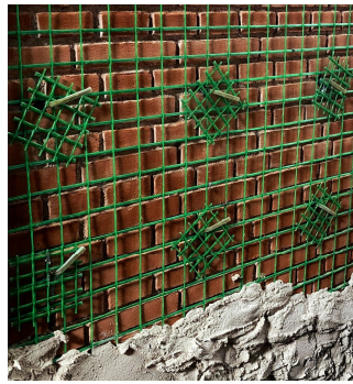
Figure 1. Application of CRM on a masonry wall.
