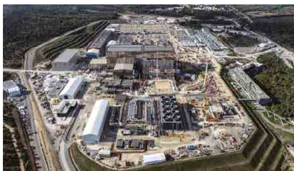
ITER building site in Cadarache, France, October 2021. Credit © ITER Organization, http://www.iter.org/
