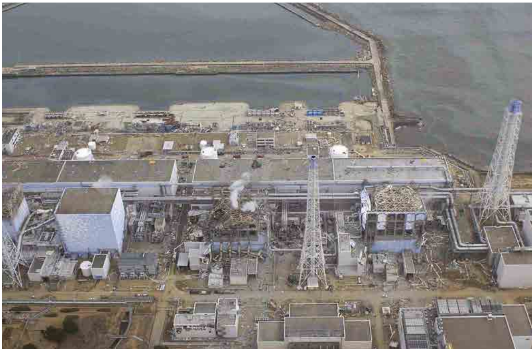
Fukushima Daiichi nuclear power plant on 20 March 2011. Aerial photo taken by a small unmanned drone. From left: Unit 1, partially seen; Unit 2, Unit 3 and Unit 4. Image credit: Air Photo Service Co. Ltd., Japan.
