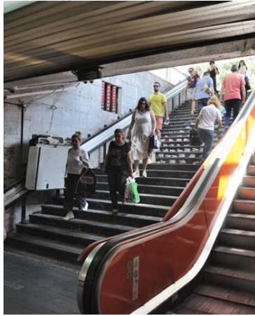
Figure 5 picture of the underground passage, bad credit rating, provided on 9/29/2022 from: https://www.novosti.rs/beograd/vesti/1031580/obnavlja-terazijski-prolaz-zavrsetku-rekonstrukcije-pothodnika-vojvode-misica-novom-beogradu-majstori-bez-predaha
