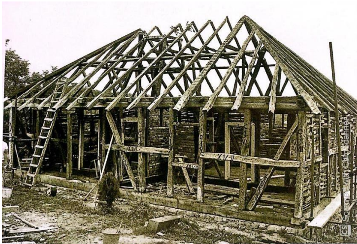
Photo 7. Photo of wooden frame structure of a Moravian house, (Pešić Maksimović, 2014)
