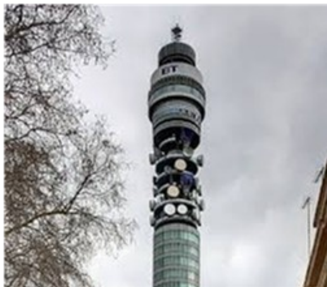
Figure 24. BT tower, Central London, location of a bank of instruments measuring the air quality in the capitol for ClearFLO
