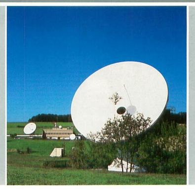
The 13.5 metre diameter antenna in the foreground and the 15 metre antenna in the background are located near Michelstadt in Germany. They ensure an uninterrupted link between Meteosat and its mission control room at ESA's Space Operations Centre in Darmstadt, Germany.
