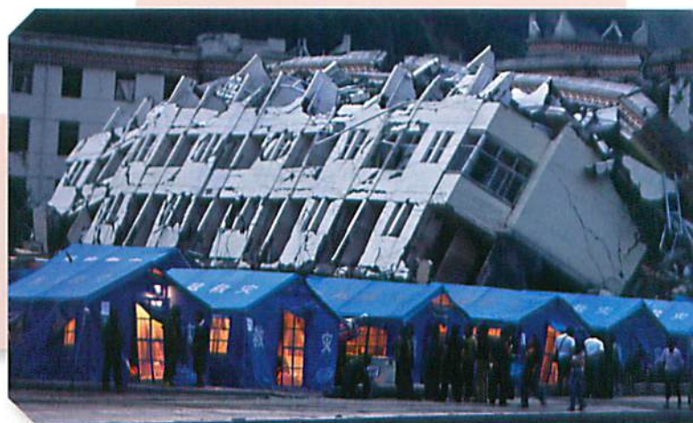
A damaged school in Sichuan province after the earthquake of 12 May 2008. Reuters/Nir Elias
