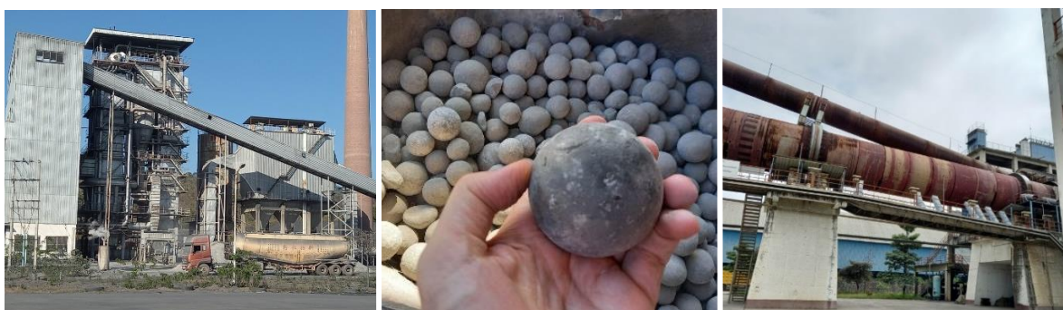
Figure 15 Coal thermal plant in cement manufacturing company with no heat recovery (left); use of ball mills for crushing clinker instead of a vertical roller mill (middle); and cement kiln without thermal insulation (right).
