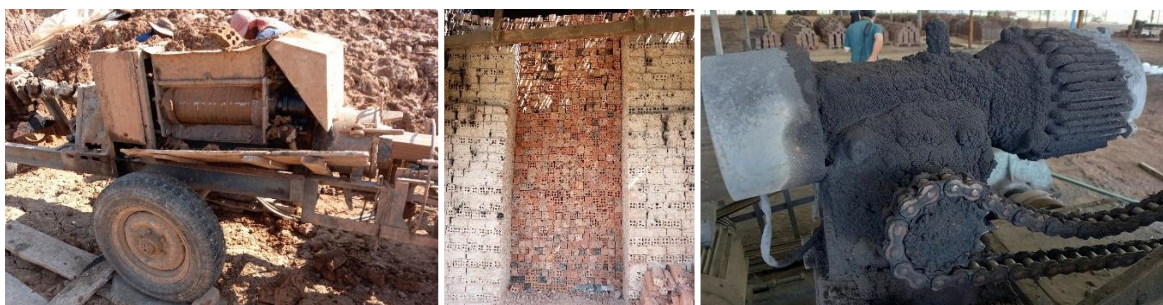
Figure 13 Use of inefficient brick-moulding machines (left) and poor thermal insulation due to the use of ordinary earth construction materials (middle); and major oil leak on mechanical transmission gearbox (right) in the brick manufacturing industry.
