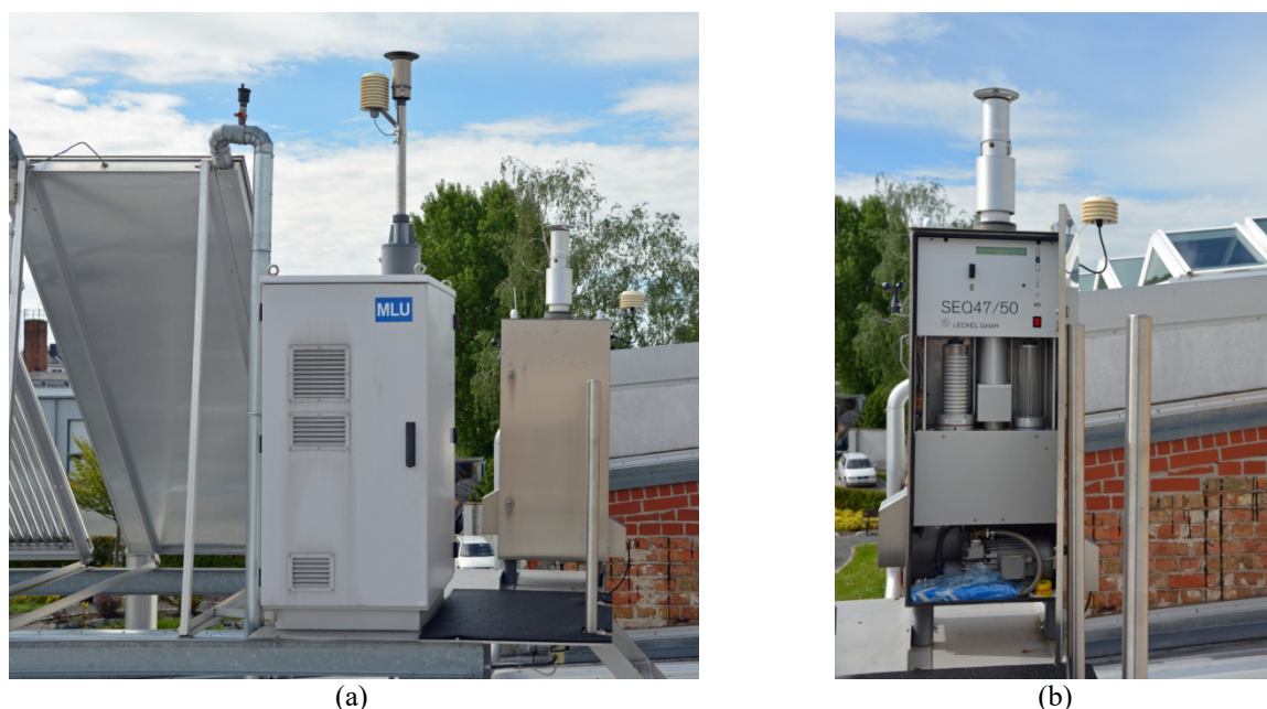
Photo 16. Sampling of air particulates in the city of Stassfurt, Germany. The equipment is installed on the roof of a house. (a) Real time particulate matter monitor 'Sharp 5030' (MLU, 2006) on the left and SEQ 47/50 Sequential Gravimetric Sampler on the right (Leckel, 2006); (b) Close-up of SEQ 47/50 Sequential Gravimetric Sampler (Source: Manfred Birke, 2015).
