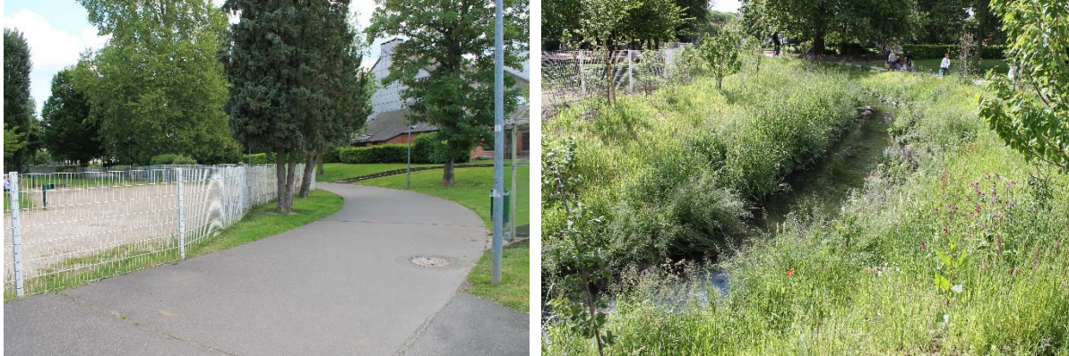
Before and after opening up the river in a densely built-up area of Sarcelles. © SIAH Croult et Petit Rosne
