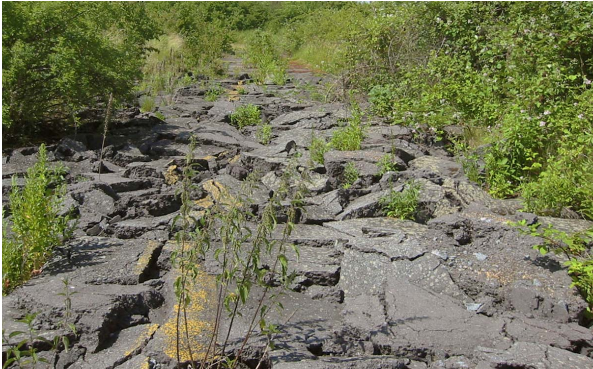
Breaking up concrete prior to natural regeneration at the former Bonames Airport (Frankfurt, Germany) © GTL, Michael Triebswetter
