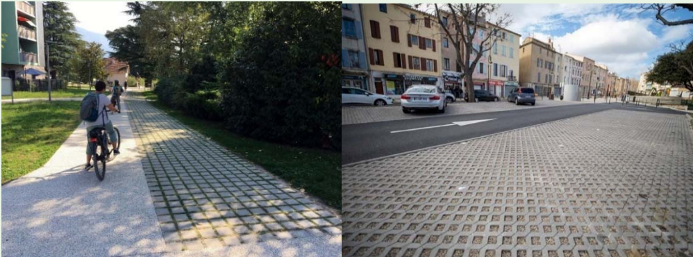
Drainage pavements or permeable asphalt, which are legitimately useful on certain surfaces to improve stormwater management, do not correspond to renaturation. ©Gilles Lecuir (on the left) ©Commune de Narbonne (on the right)
