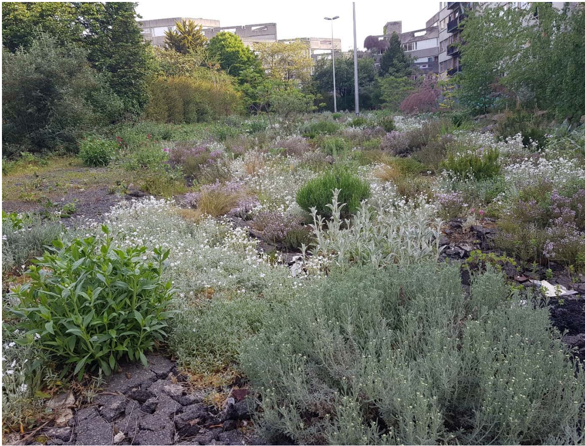
Concrete crushing and planting on a former parking lot in the city of Aubervilliers, France ©Wagon landscaping
