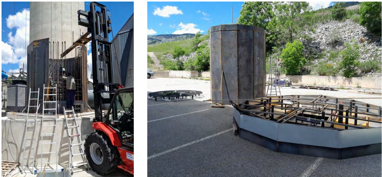
Figure 11: Assembly of inner and outer formworks for the wall [20/06-09/07/2022]
