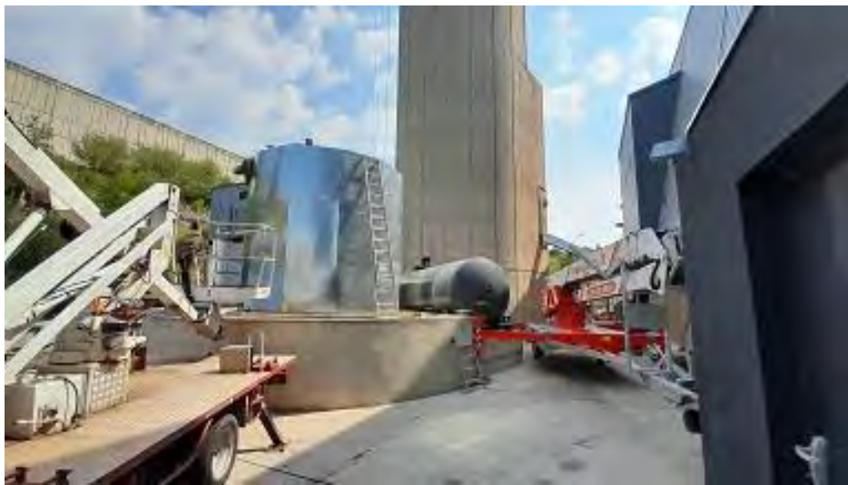
Figure 17: Installation of a crane at THEMIS site [16/08/2022]
