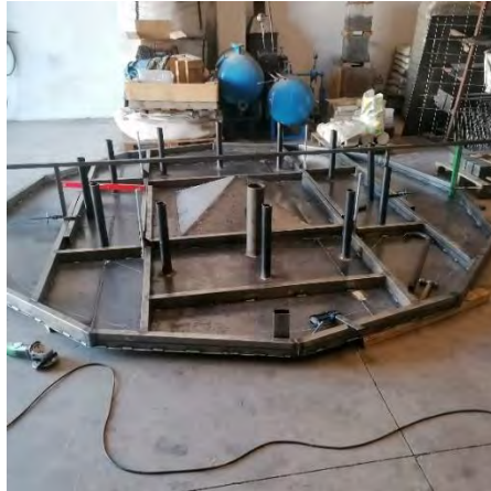
Figure 4: Construction of top cover of tank in Spain [15-19/11/2021]
