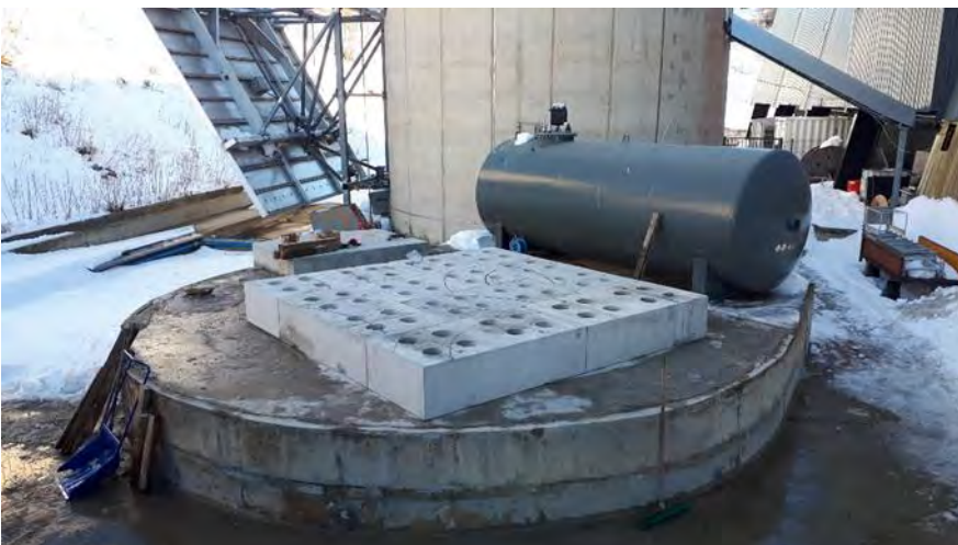
Figure 6: Assembly of TES basement and Implementation of TCs in the basement [13-17/12/2021]
