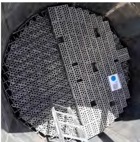
Figure 18: Installation of filler bricks and implementation of the instrumentation (TCs) [17-31/08/2022]
