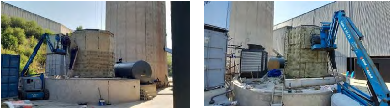
Figure 14: Installation of the outer thermal insulation [19/07/2022]
