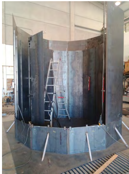
Figure 8: Construction and pre-assembly of the formworks of the wall in Spain [09-13/05/2022]
