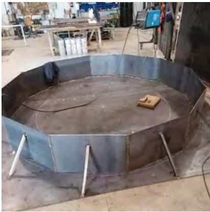
Figure 2: Construction of bottom formwork (left) and intermediate grids (right) [01-05/11/2021]
