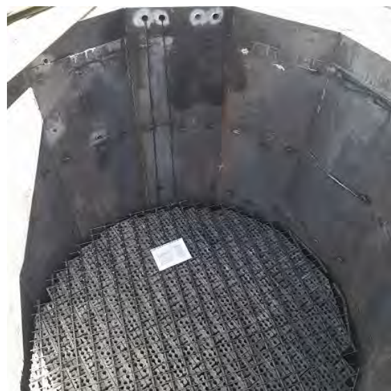
Figure 18: Installation of filler bricks and implementation of the instrumentation (TCs) [17-31/08/2022]
