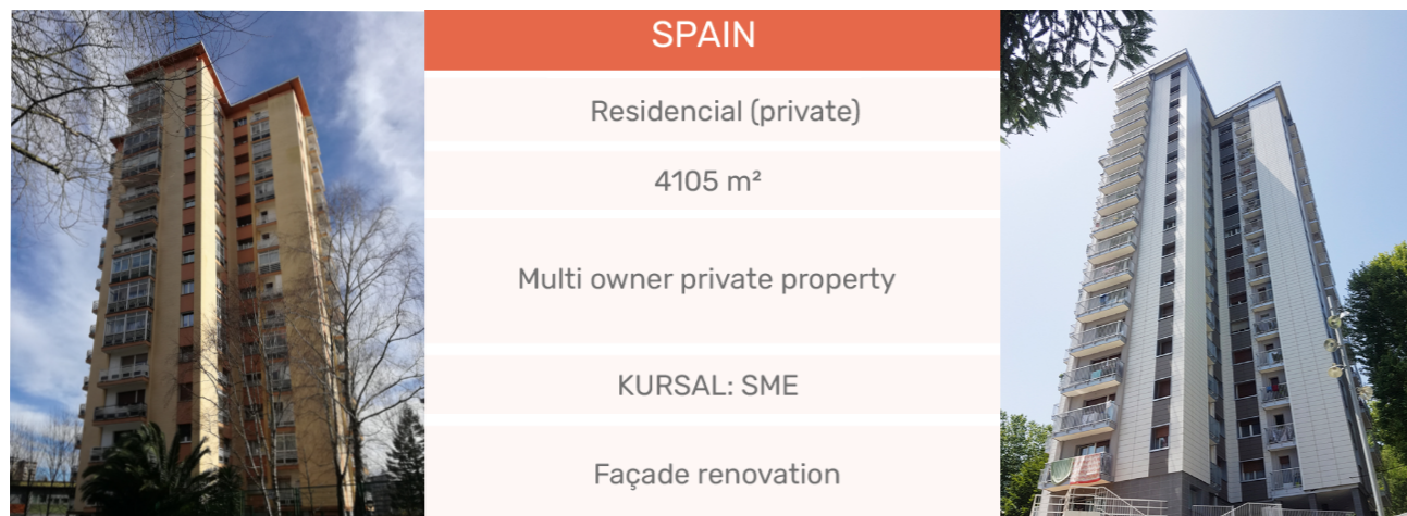
Figure 11 : Use case in Spain: façade renovation in a private residential building
