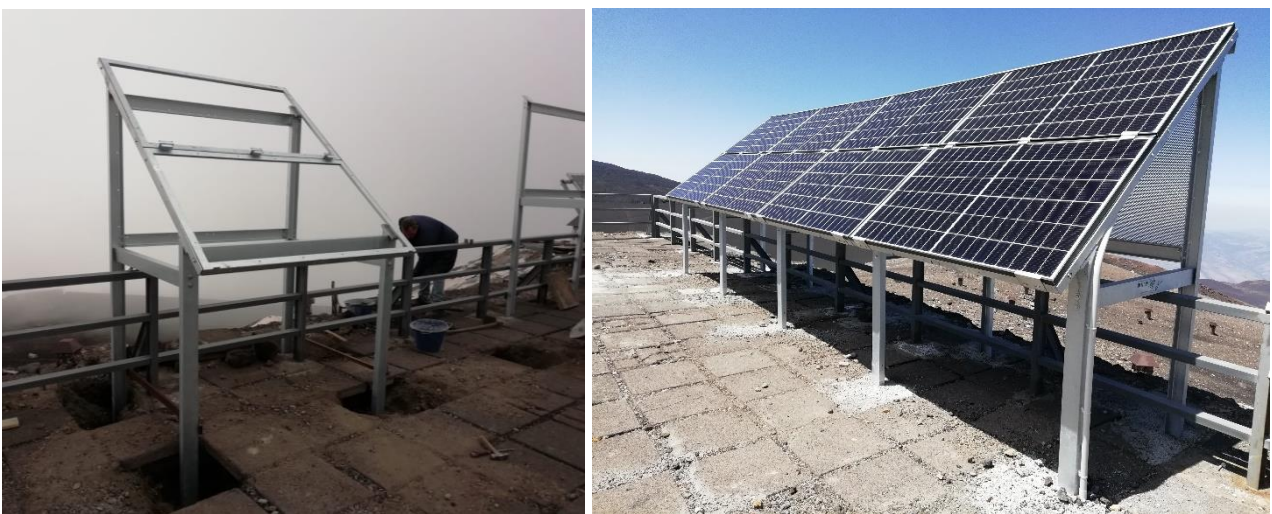
Figure 3 – Left: a phase of installation of the galvanized-iron solar panel structure at PDN on 9 July. Right: the structure after completion of the installation, with eight 350 W photovoltaic panels mounted on it.
