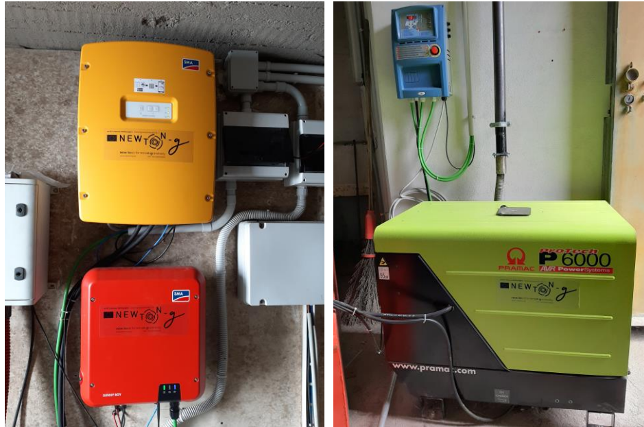
Figure 4 – Components of the off-grid power system installed at PDN. Left: battery management system (SMA Sunny Island), in yellow, and photovoltaic inverter (SMA Sunny Boy), in red. Right: diesel generator.
