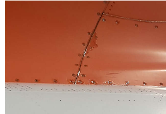
Paint line erosion of a Vertical Tail-Plane (A320)
