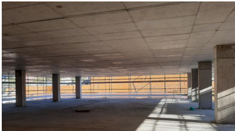
Figure 19: Finished concrete columns
