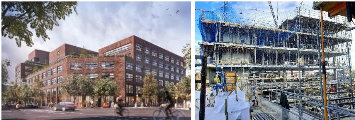
Figure 13: MILE office building as a rendered image (Provided by BIS structure) and during construction
