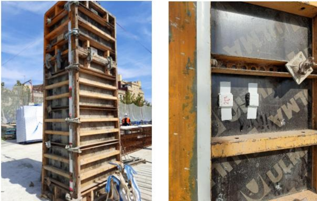
Figure 18: Concrete column formwork with installed accelerometers at demo# 6
