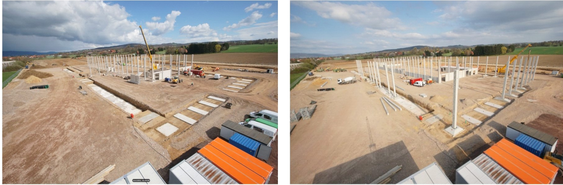
Figure 17: Time-lapsed images from Rinteln construction site (Goldbeck 2021)
