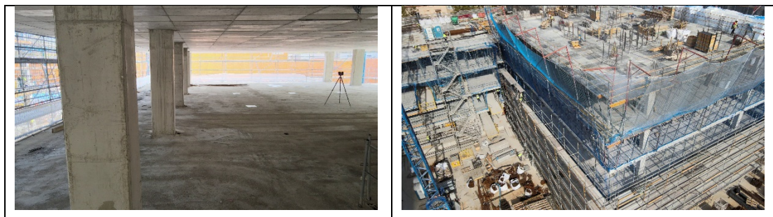
Figure 10: Demo Site #6 construction site a) indoor and b) outdoor drone recordings.
