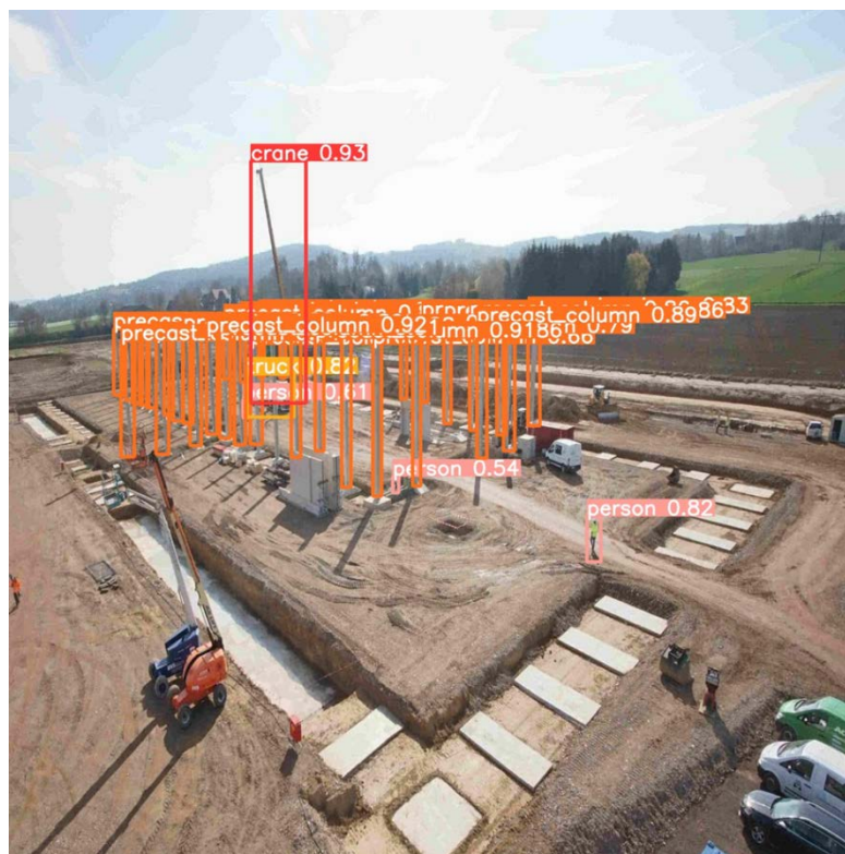
Figure 36: Site object detection example 2
