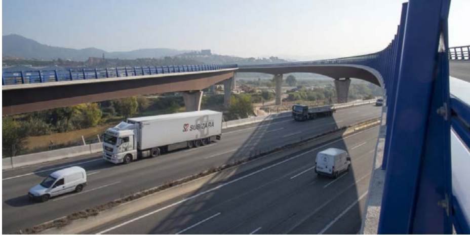
Figure 9: Bridge of Demo Site #7 construction.
