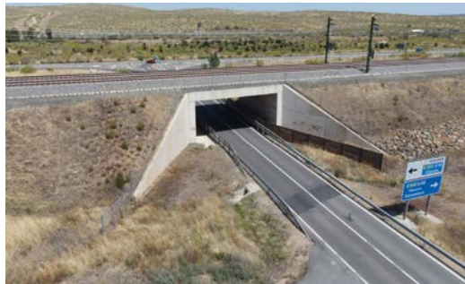
Figure 8: Demo site #1 : Underpass located at the 3 + 93 PK.
