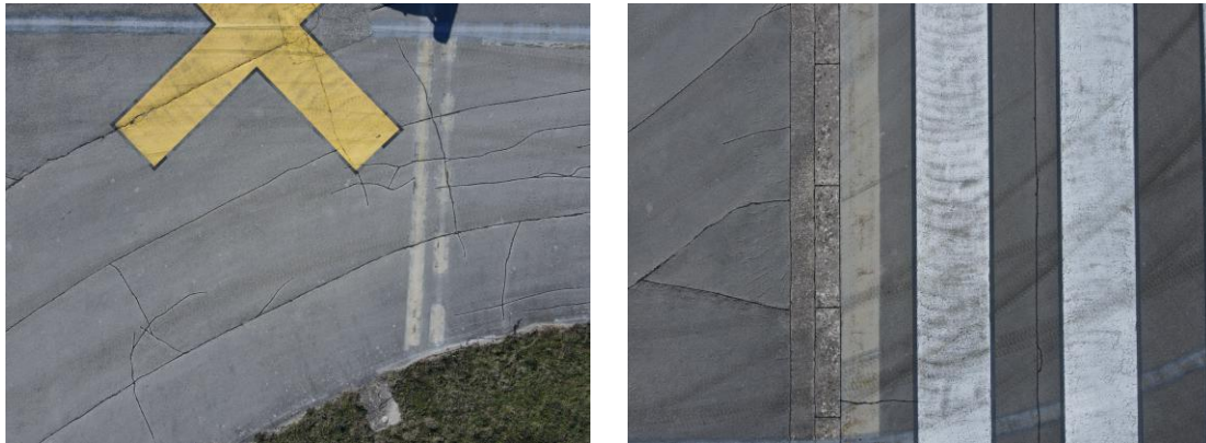
Figure 5: Data via UAV camera of Zadar airport
