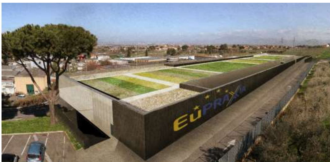
Fig 9: 3D-rendering of the EuPRAXIA construction site at INFN-LNF. The design process of the building has recently started, it will have dimensions of 134m x 35m with a potential extension added at a later point (image credits: Simona Incremona, General Services and Technical Division).
