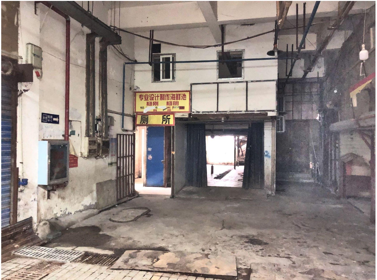
Supp. Fig. 1. Looking West along 5th street. Male and Female toilets entrance below yellow sign at left rear of image. WHO Mission (2021).
