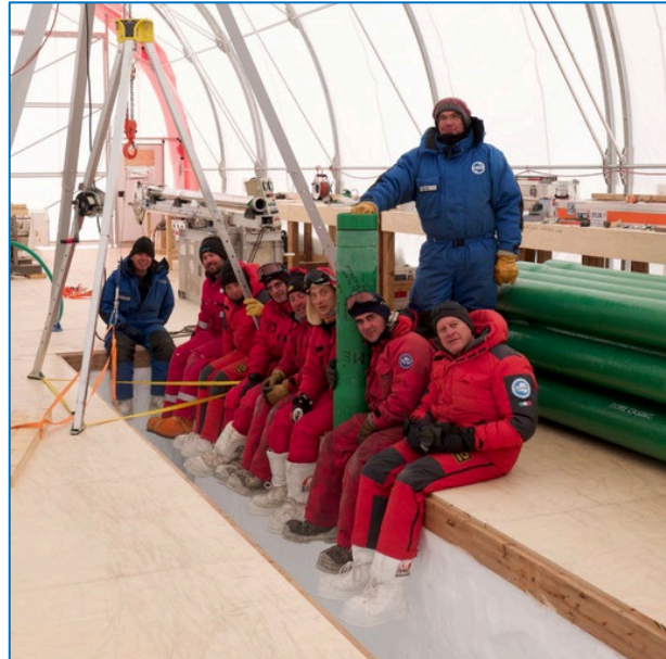
In preparation of the casing operation at the BEOIC drilling trench (Credits: Carlos Barbante ©PNRA/IPEV)
