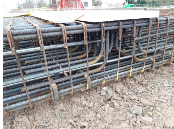
Figure 6. Cage with foamboard attached.
