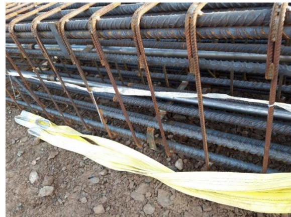
Figure 5. Wire placement in the cage.
