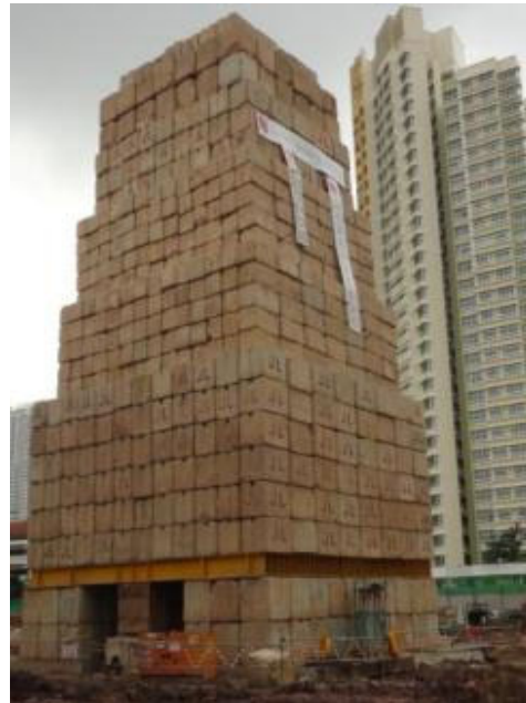
Figure 1. Massive Kentledge Test by Stacking Concrete Blocks
