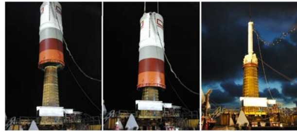
Fig. 10. The installation of a 6.5 m pile with the use of a Noise Mitigation Screen (IHC Offshore Systems) at the German offshore wind farm Riffgat in the North Sea. In the left and middle pictures, the NMS is positioned by the crane around the monopile. In the right picture, the hydraulic hammer is positioned at the head of the pile and the NMS is invisible. Source: Author's personal archive from the Riffgat Offshore Wind Farm (2012).
