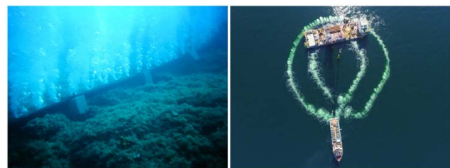
Fig. 7. (Left) Air-bubble cloud released by a perforated pile positioned on the seabed. (Right) Double Big Bubble Curtain (DBBC) deployed around the Giant7 floating piling vessel in the Winger OWF, Germany. Source: © Hydrotechnik Lübeck GmbH ( https://www.hydrotechnik-luebeck.de/blog/portfolio-item/0003-borkumwest2-00/ ).
