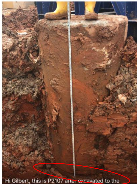
Figure 15. Photo of excavated pile head showing the horizontal crack (Case 4, Site E).
